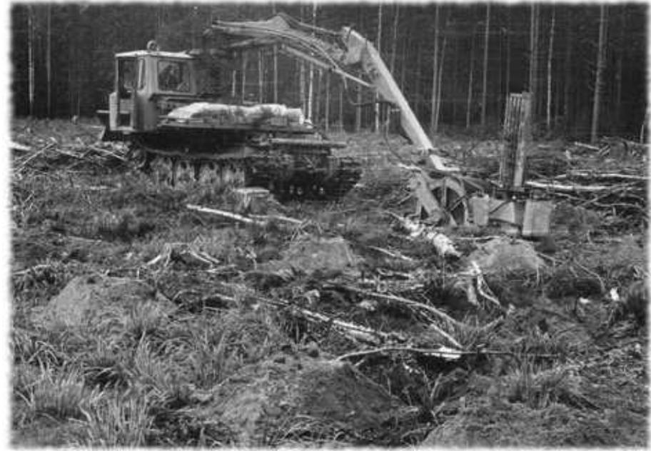
Container seedling planting machine "KLM-1" (Russia) mounted on excavator "TB-1" able to make mound and simultaneously plant seedling on it 1983.
